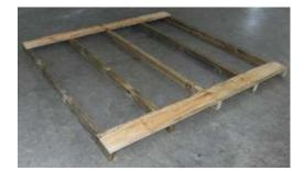
Step 2: Lay out remaining floor boards. Measure diagonals to ensure measurements are equal (I.e. floor is square). Rip down last floor board to suit gap, and nail off floor with 50mm flooring nails (10 nails per board).
